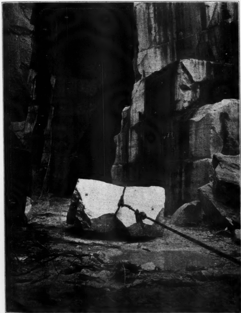
Block of Marble Being Pulled Horizontally By Means of the Top Derrick to the Opening
